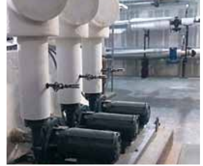
Pictured at top: High Rise Building, Mexico City, MX. Pictured in the middle and at bottom: Texas Children's Hospital, Houston, TX.
